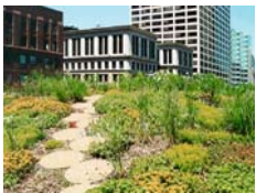
Improving the city climate, greening of roof surfaces also significantly reduces rainwater run-off through detention, storage and evaporation of the rainwater.
