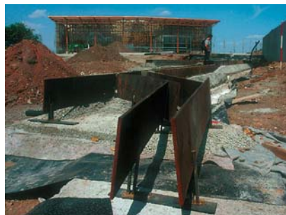
The water fissure under construction, showing the steel structure of the foundations. The Academy is in the background, with the largest solar roof in Europe.
