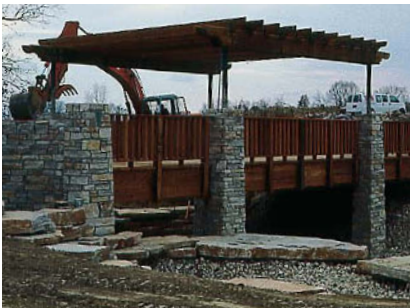
Pedestrian bridge under construction
