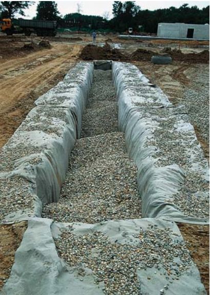
Constructing a swale system between parking spaces
