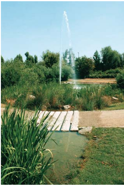
The stream runs through a purification biotope into the aerated retention pool.
