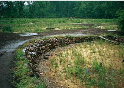
The sewage seeps through several planted tanks and harmful substances are removed by organic decomposition processes at the various purification stages.
